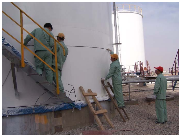
Figure 1. Picture of work in soralchin adrar
